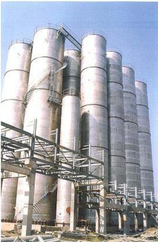
18 NOS. S.S. 304 STORAGE TANKS DIA. RANGING FROM 3.2 TO 6.5 M AND HEIGHT OF 20 TO 35 M, TOTAL 761 MT FOR M/S. VVF LTD., FATTY ACID PLANT AT TALOJA, UNDER UHDE INDIA LTD., INSPECTION.
