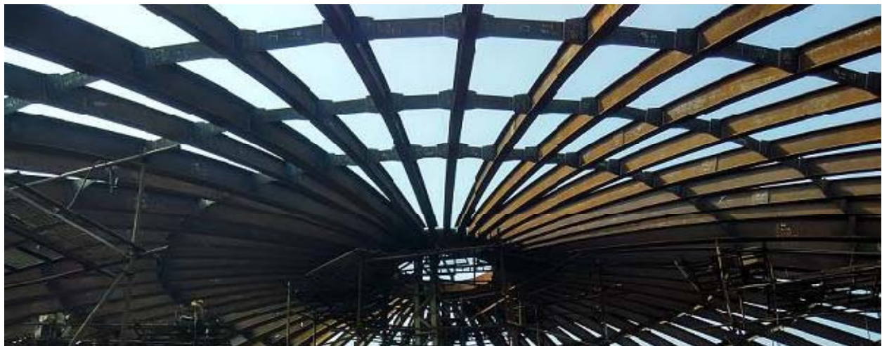
RAFTER AND CROSS GIRDER ERECTION
