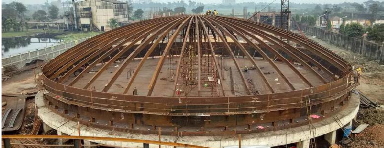
ERECTION OF MAIN RAFTER
